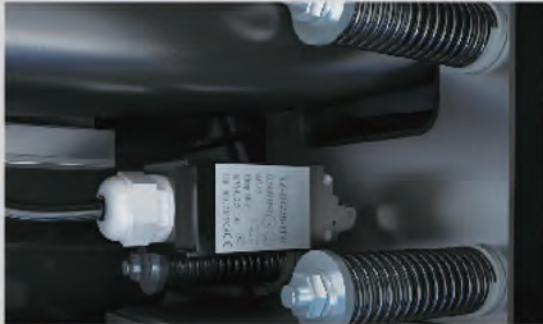
Handrail inlet protection device
